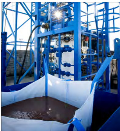
Tore Scrub Sand Handling System
