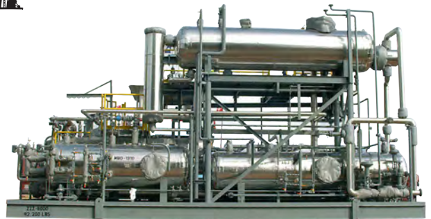
Gas Dehydration Unit
