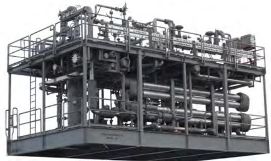
Fuel Gas Conditioning Unit
