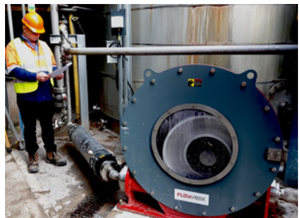
Flowrox LPP-T pump with 80 mm Flowrox Expulse™ stabilizing the flow in a filter feed application.
