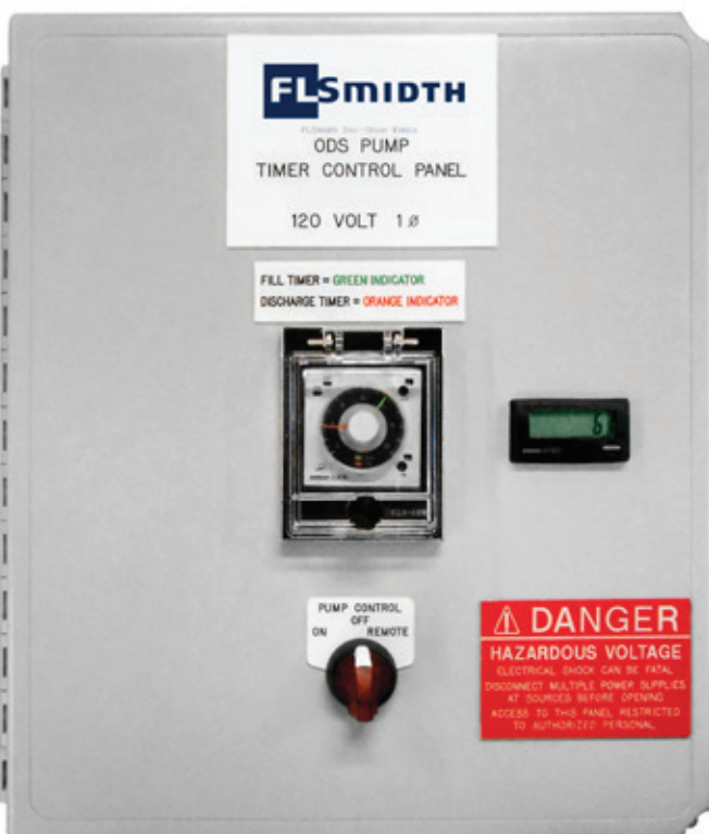
Pump control panel with adjustable, variable timer.
